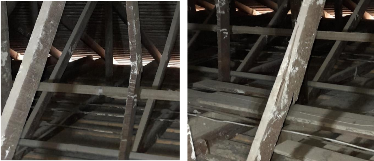
Figure 2 and 3: Showing Web member of the truss that are damaged
