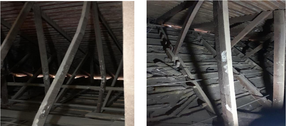
Figure 4 and 5: Showing damaged web members
