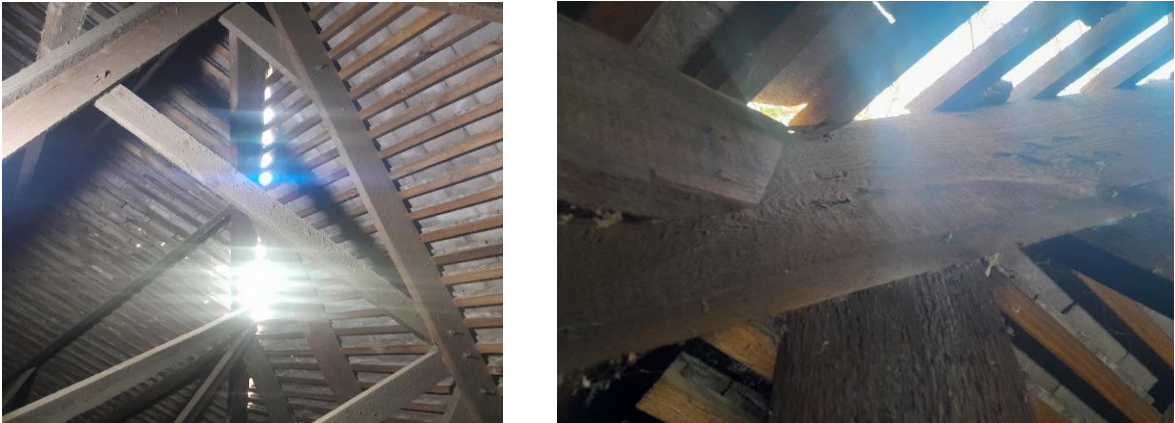
Figure 4 and 5: Showing damaged web members
