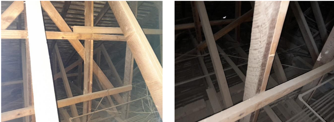
Figure 6 and 7: Showing laminated member in the roof
