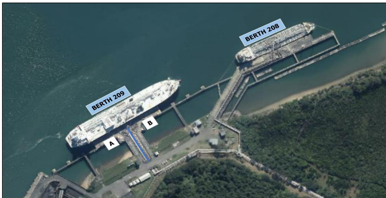
Figure 2: Berth 208 & 209 at the South Dunes precinct
